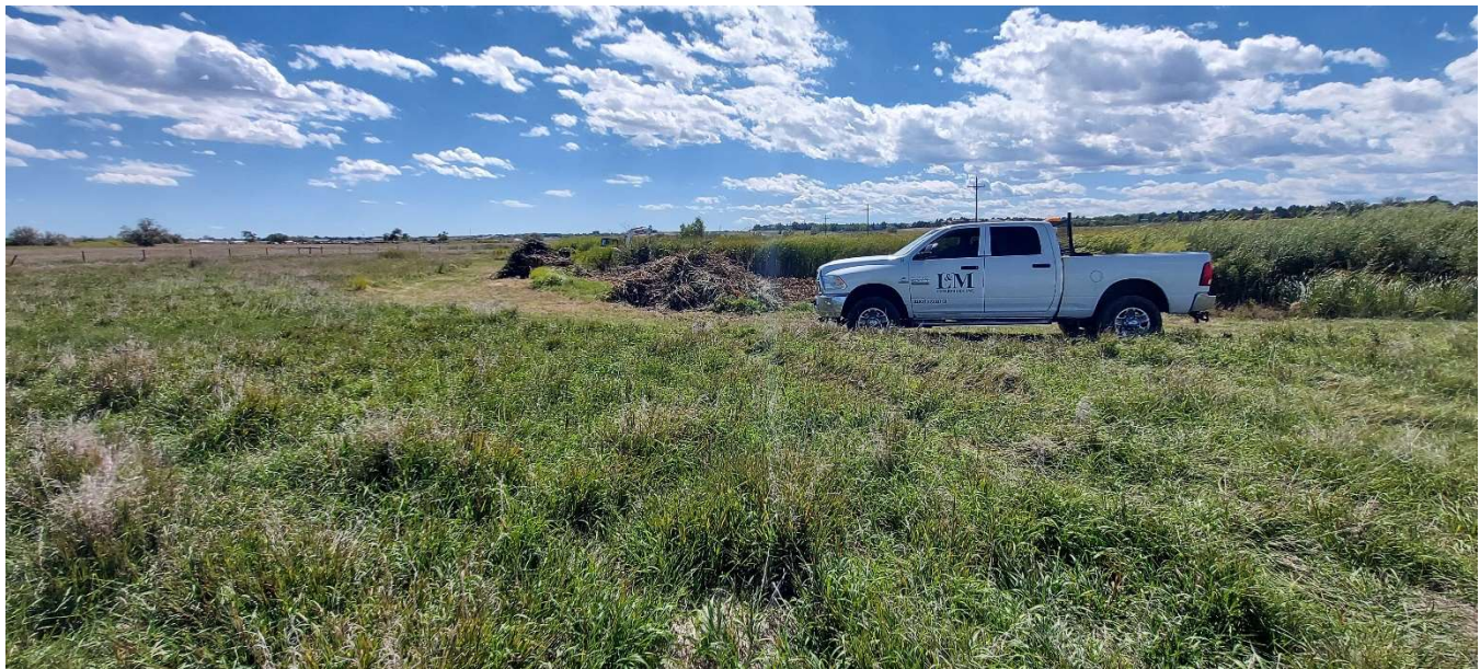
Photo – Contractor working on Priority 2 Site
