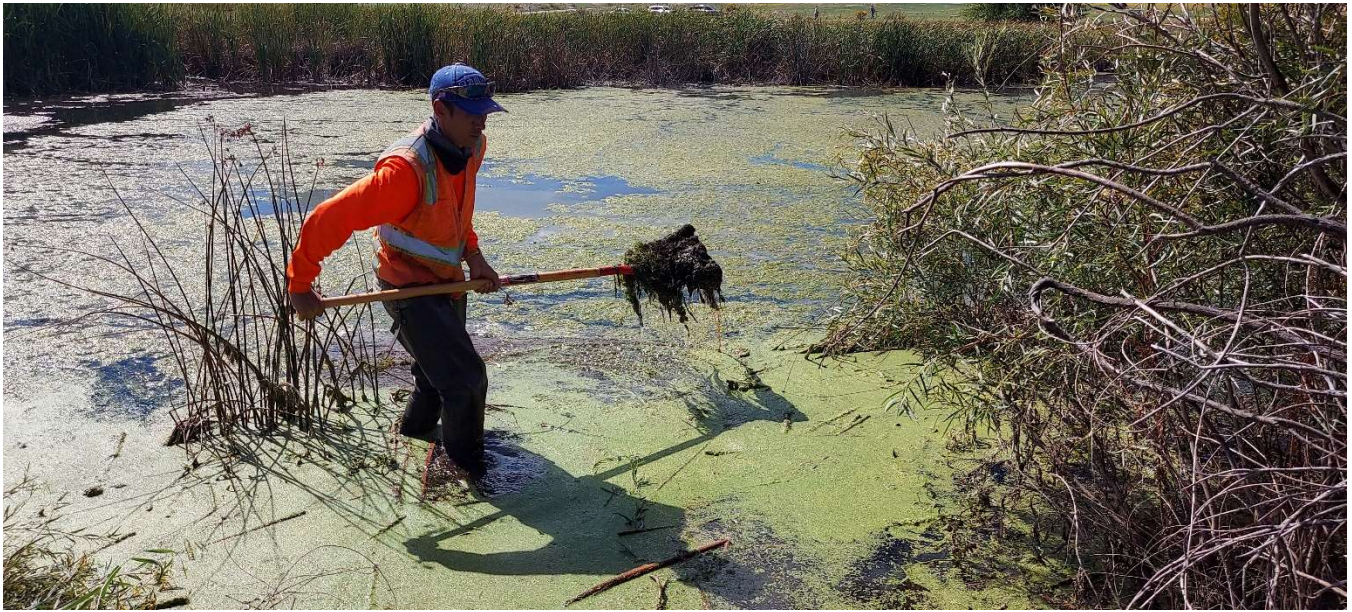
Photo – Contractor cleaning out Peoria Pond Outlet Grate
