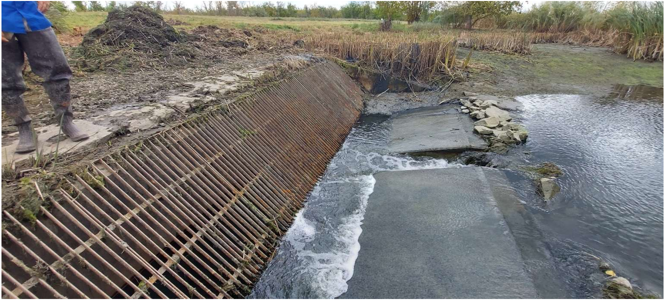
Photo – Peoria Pond Outlet Grate after cleaning
