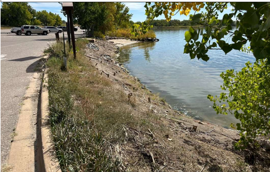
Reseed and mulch 2022 maintenance project.
