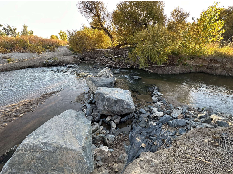
Severe erosion at breakout area
