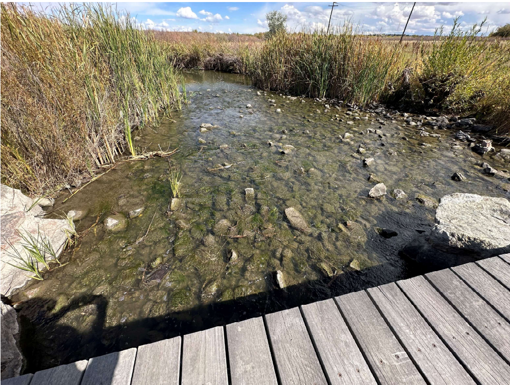
Riffle structure at lower trail crossing
