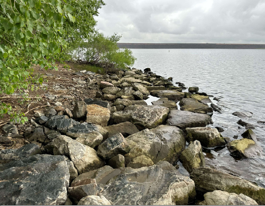
Current condition of shoreline stabilization
