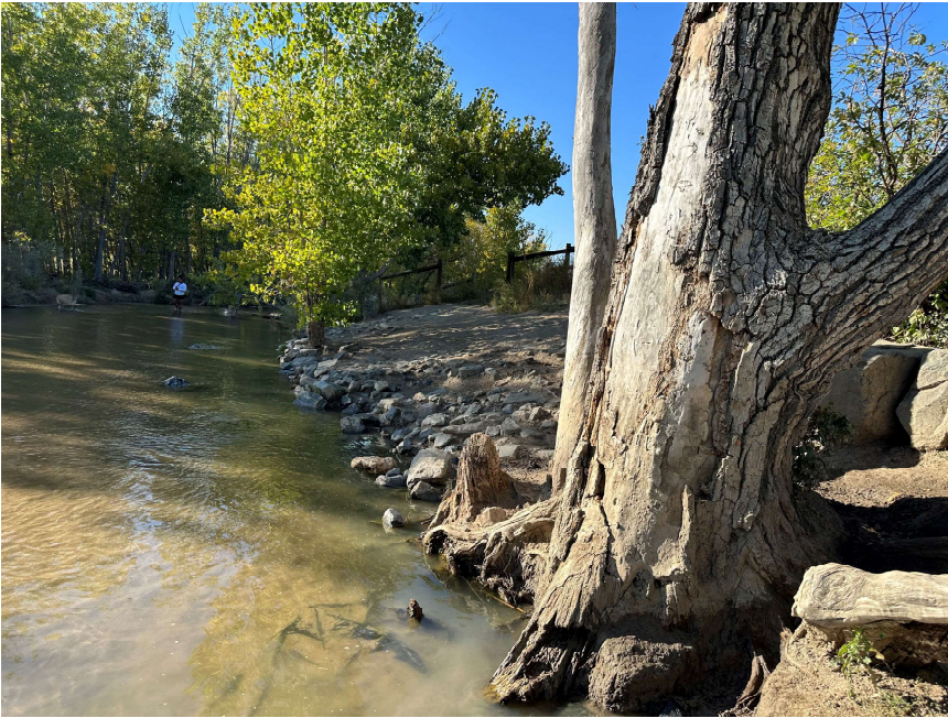
Boulder edging erosion below Access 4. Also note in-stream sediment deposition almost to the level of the original boulders.
