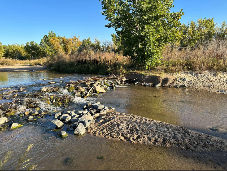
Grade control structure continued to work well
