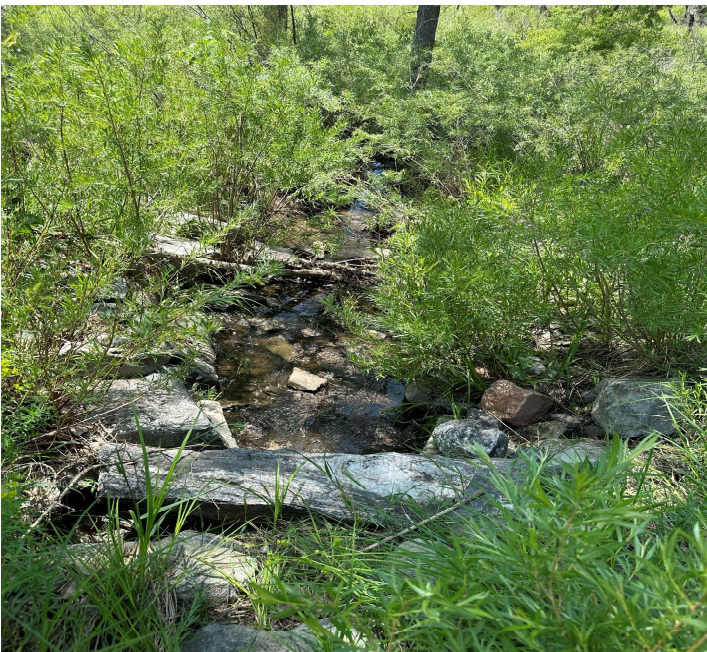
Outlet of the outlet structure
