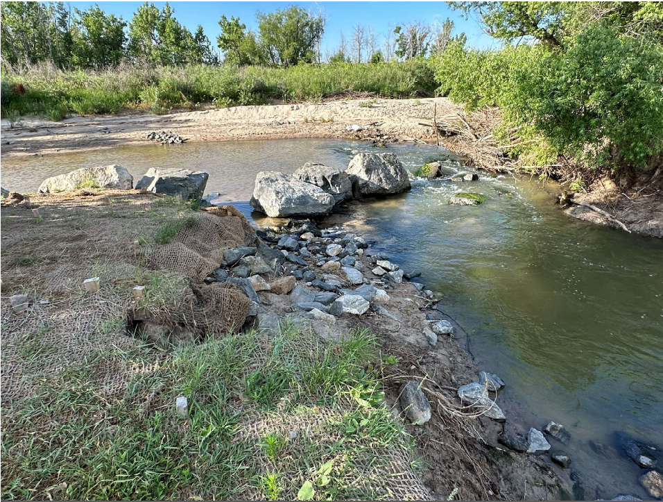
Severe erosion at breakout area
