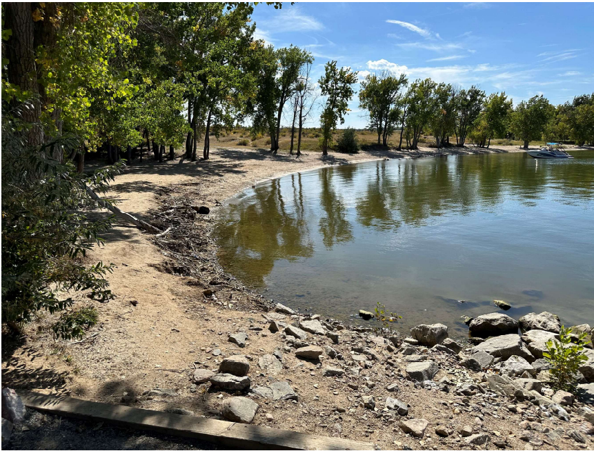
100-foot eroding shoreline that will be stabilized by current maintenance project.
