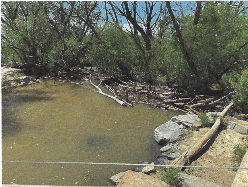
Photo 16- Boulder erosion at Access 6
