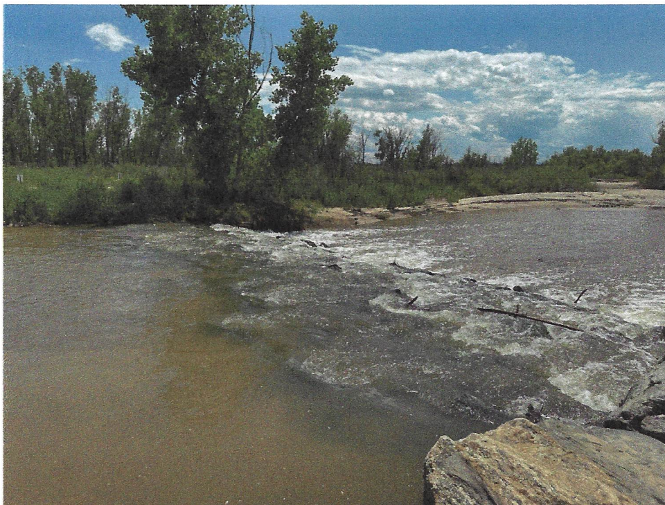
Photo 21- Grade control structure worked well
