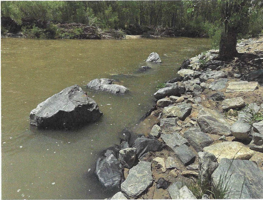
Photo 15-Boulder edging erosion
