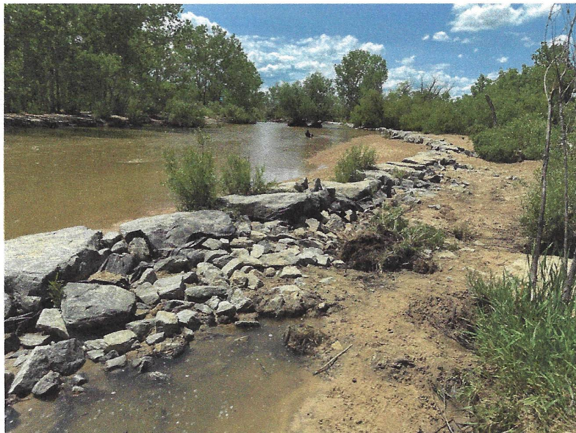
Photo 18-beginning of beach area- severe erosion behind the boulder edging and of the beach itself
