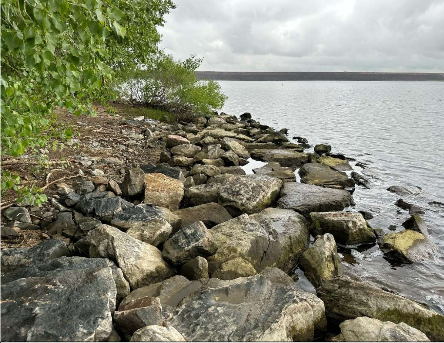
Current condition of shoreline stabilization
