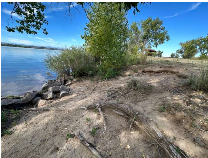
Flood caused above stabilization level erosion
