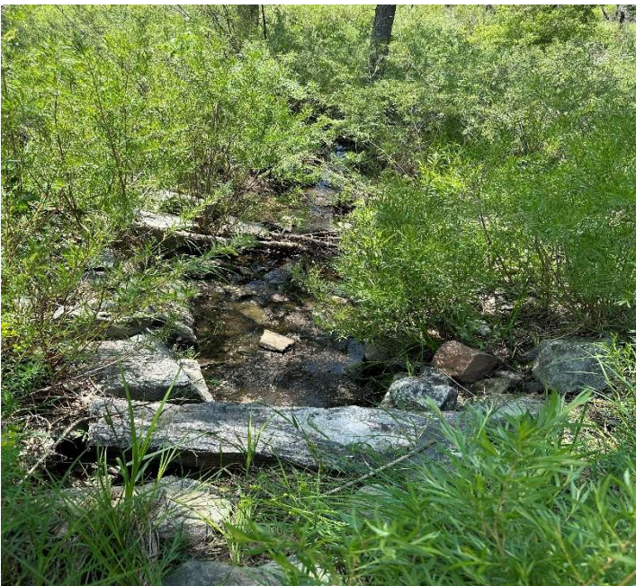
Outlet of the outlet structure
