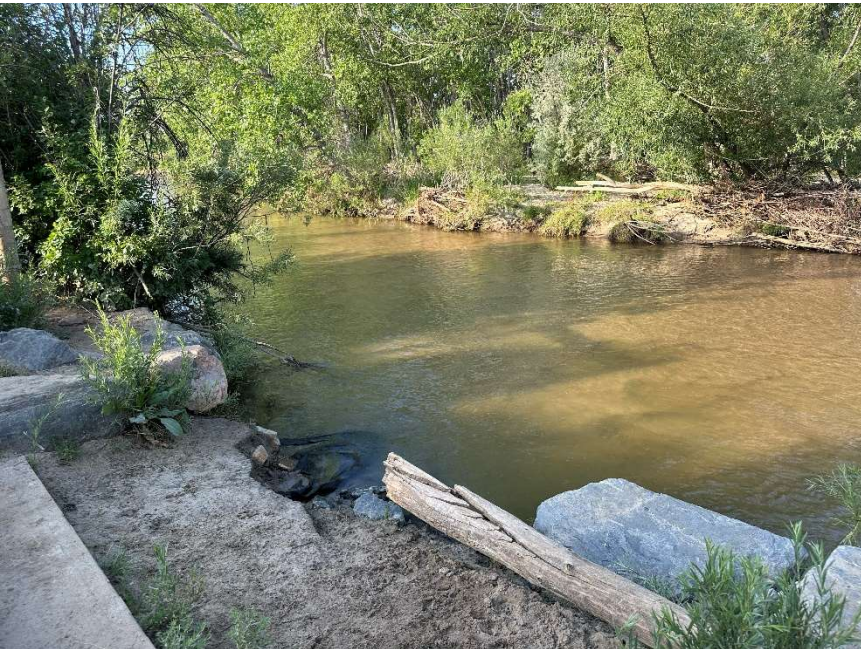
Boulder erosion at Access 6
