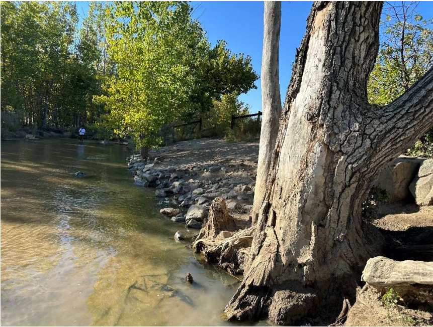
Boulder edging erosion below Access 4. Also note in-stream sediment deposition almost to the level of the original boulders.
