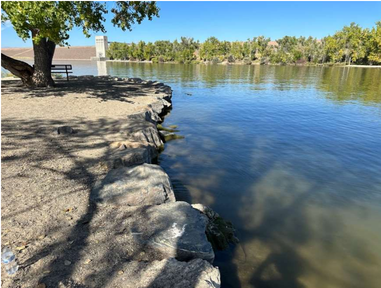
East Shore of Stabilized area
