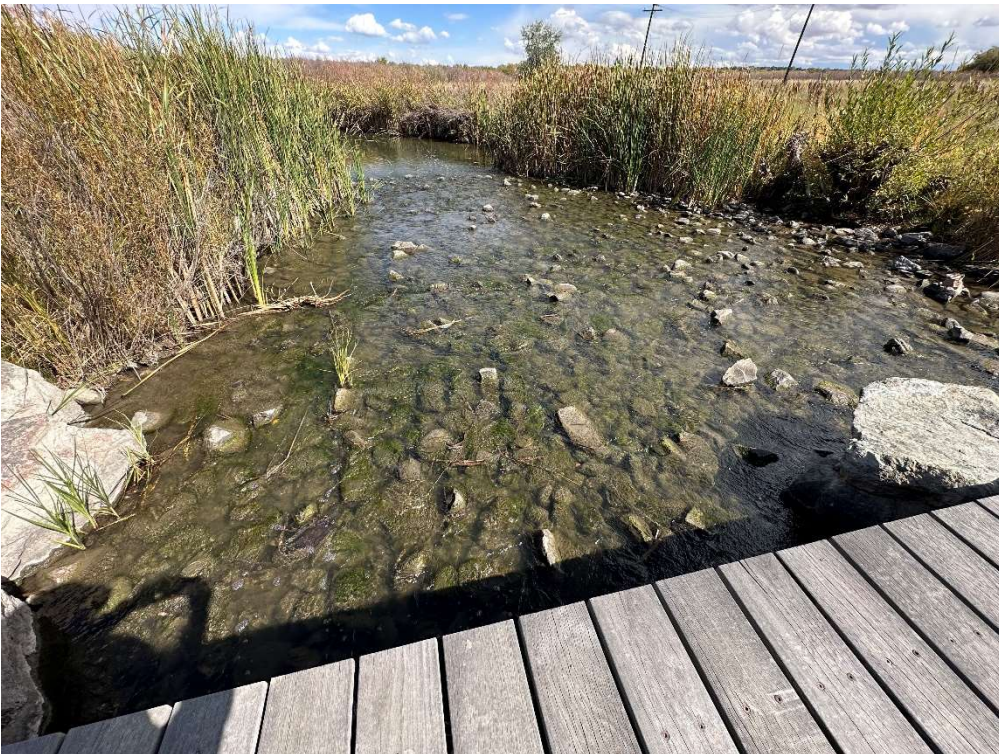
Riffle structure at lower trail crossing
