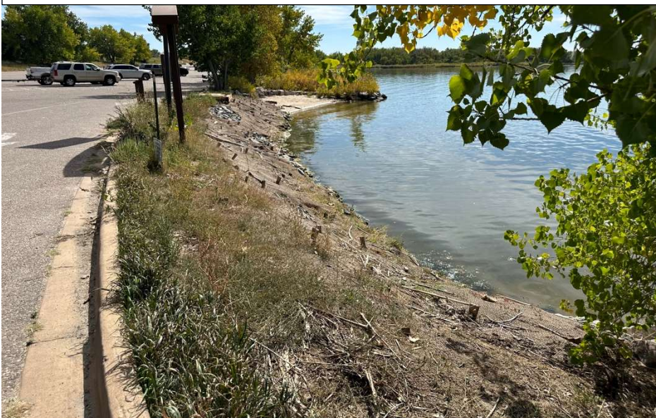
Reseed and mulch 2022 maintenance project.
