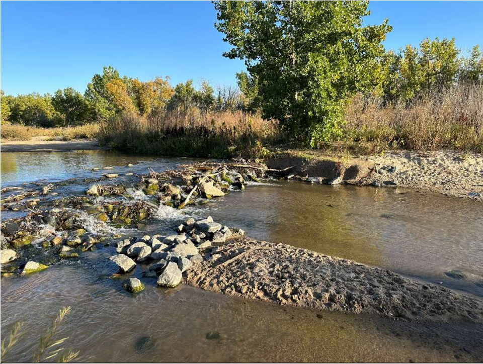
Grade control structure continued to work well
