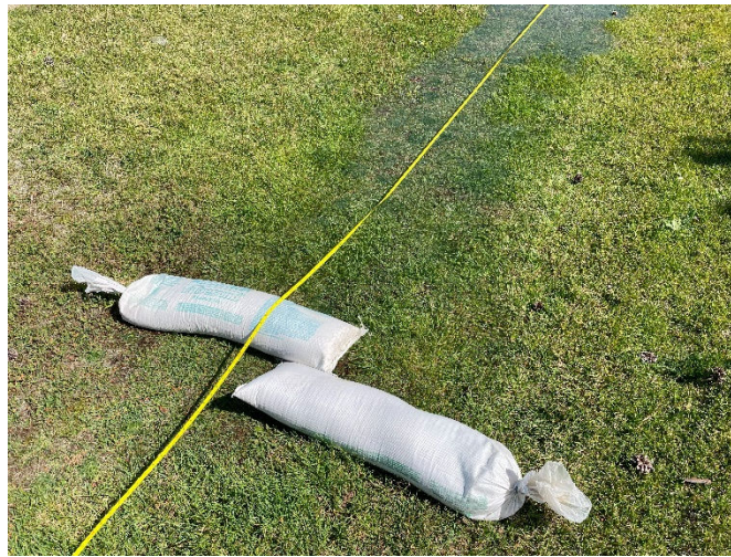
Figure 13. Two sandbags placed end to end functioned as check dams during the third and fourth SRTs at RoadSafe
