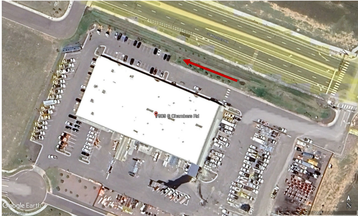
Figure 12. RoadSafe site with combination grass buffer and grass swale with red flow direction arrow (Google Earth image)
