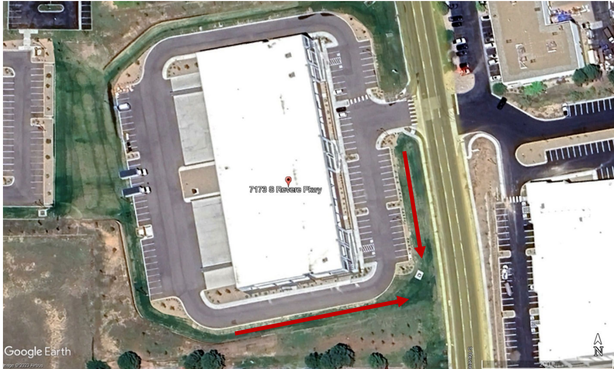
Figure 18. Central Centennial industrial building with two swales draining to single outlet structure (Google Earth image)
