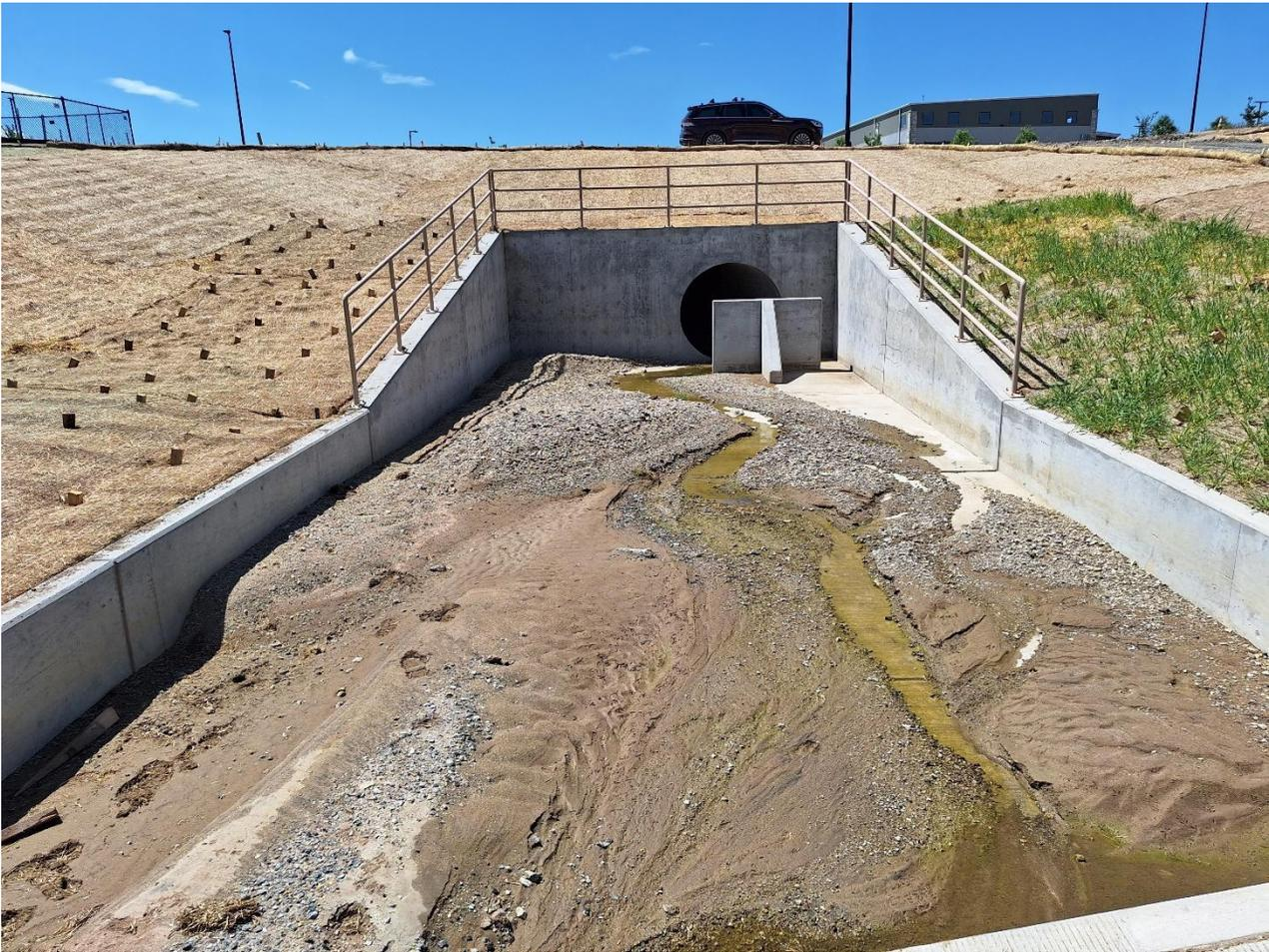
Photo of Dove Creek Phase 1 construction completed sediment capture area downstream of Otero Avenue
