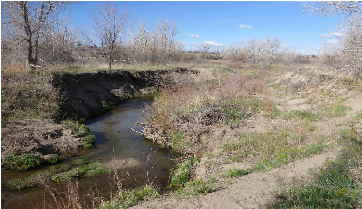
Photo of Piney Creek in Cherry Creek State Park (courtesy of Muller Engineering)
