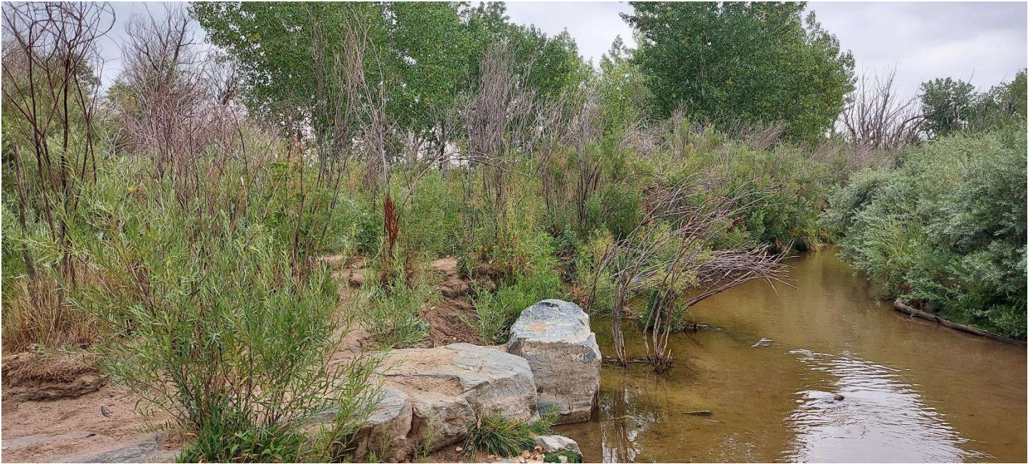
Photo 23 (Bank Erosion on 7/28/22)
