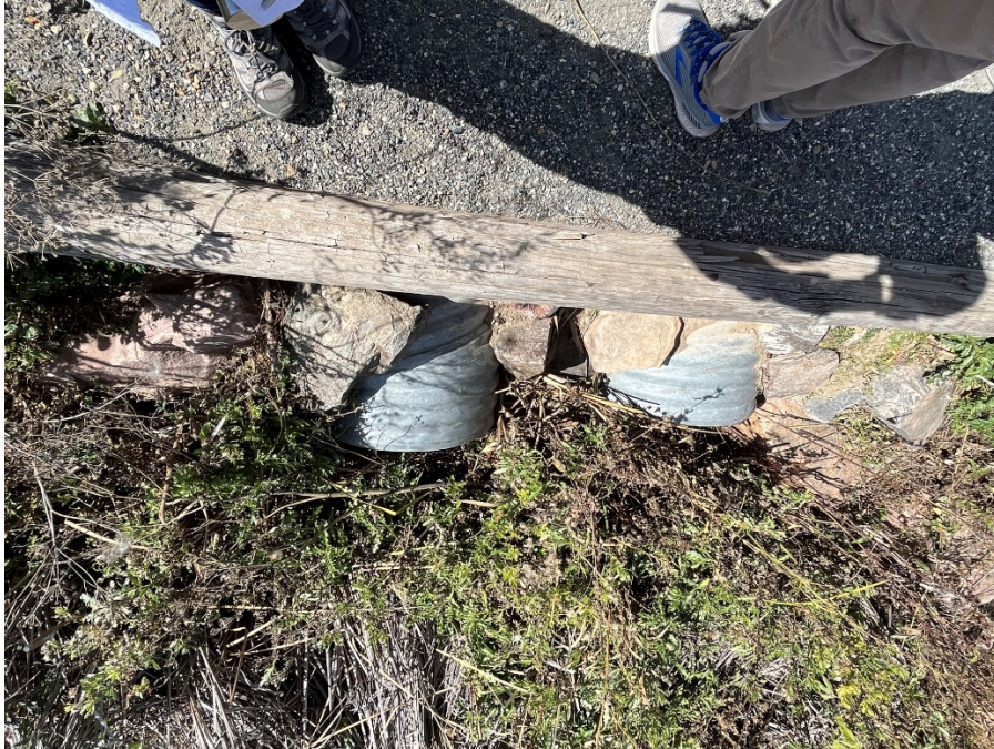
Photo 8. Existing CMP culvert for Windmill Creek under gravel road.
