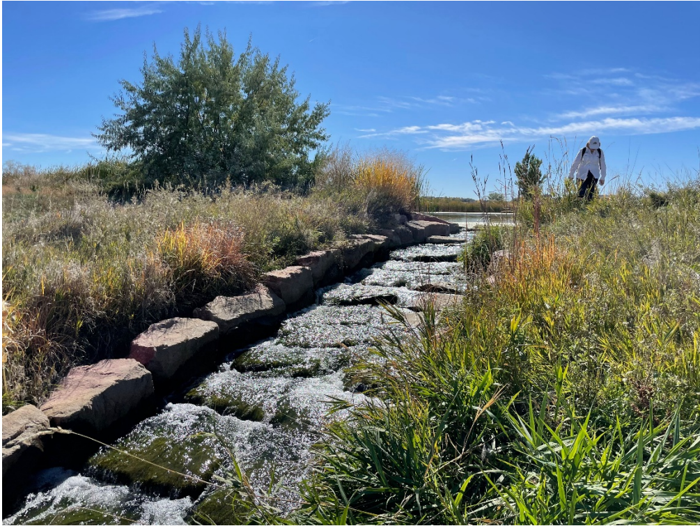
Photo 12. Lone Tree Creek Pond outlet structure and upper portion of rundown
