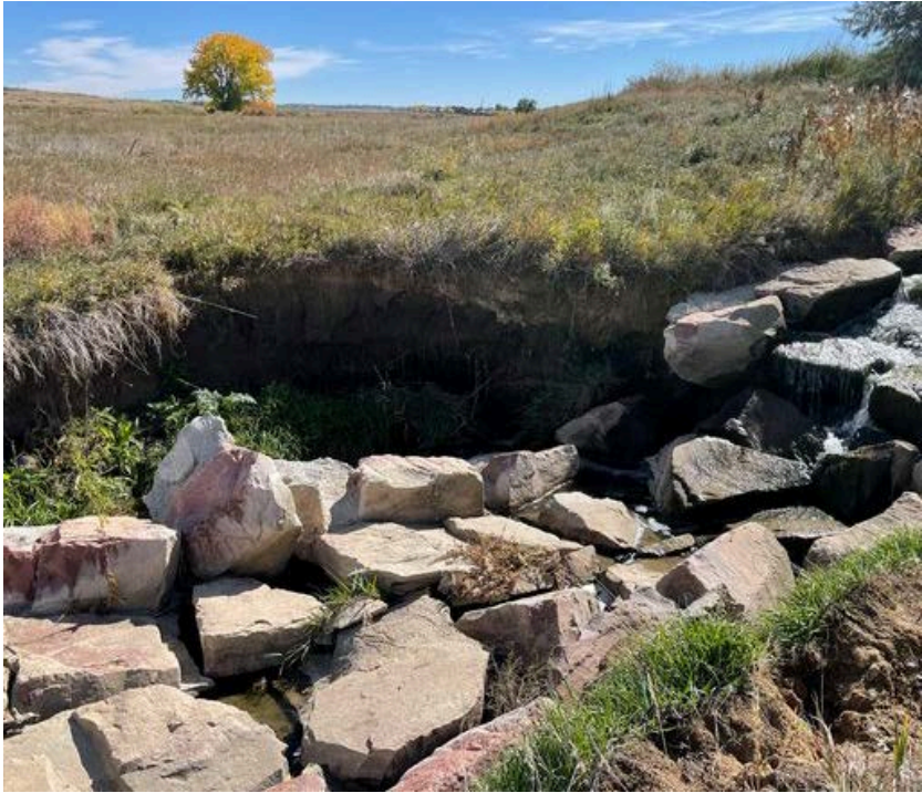
Photo 14. Channel erosion along Lone Tree Creek below Lone Tree Creek Pond.
