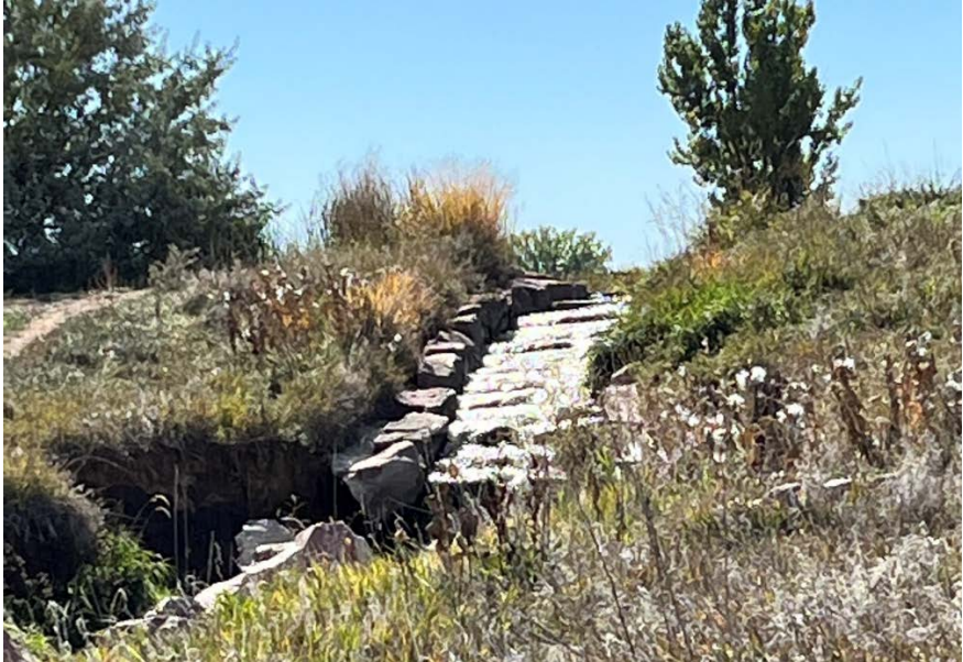
Photo 14. Channel erosion along Lone Tree Creek below Lone Tree Creek Pond.
