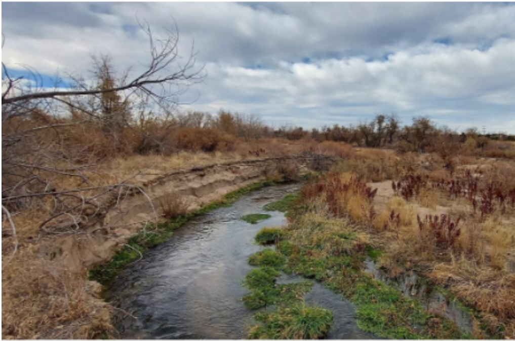
Figure 2: Bank Erosion Downstream of Arapahoe Road
