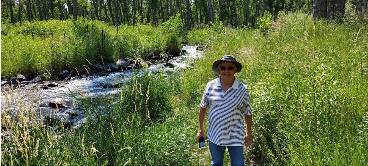
Cherry Creek – Sheetpile and riprap protection for Aurora Waterlines (Photo from 7/15/21 Field Trip)
