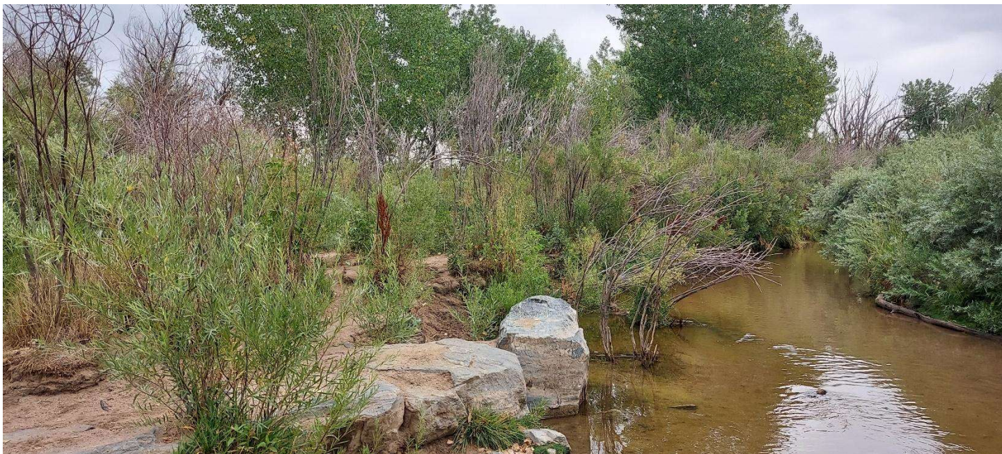
Photo 23 (Bank Erosion on 7/28/22)
