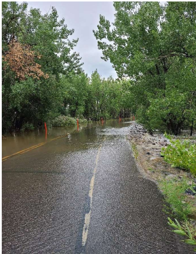
Storm Photo - Cherry Creek at Lake View Drive
