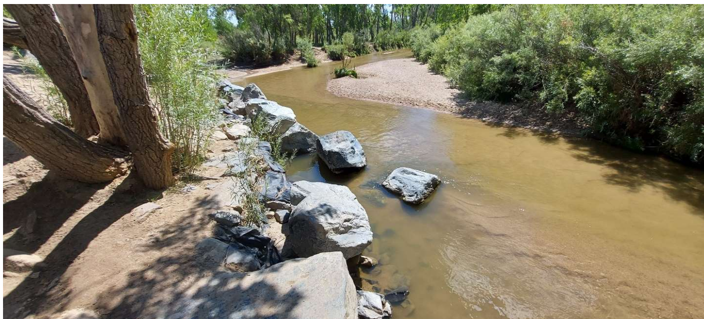
Photo 30 (Bed and Bank Erosion at post-storm visit on 8/23/22)
